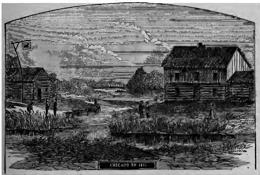
PRESENT SITE OF LAKE STREET BRIDGE.
