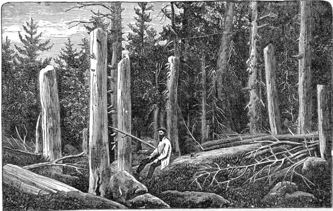
Starvation Camp.—Stumps cut by the Donner Lake Party, 1846. For full description see page 167. (From photograph by Thos. Houseworth & Co., San Francisco.)
